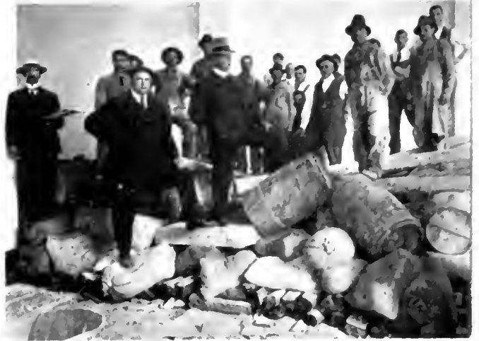
Fig. 2—Concrete test. Curry Building, Winnipeg, Man.
